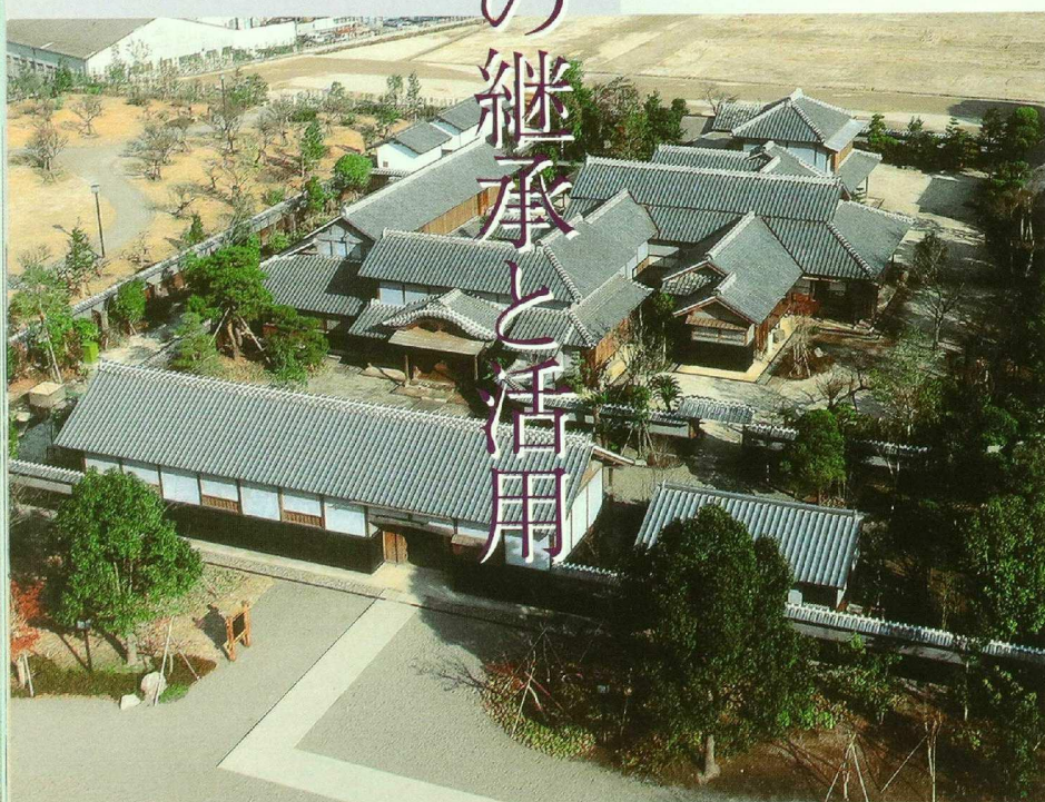
旧細川刑部邸 Former Hosokawa Gyobu-Tei Residence
